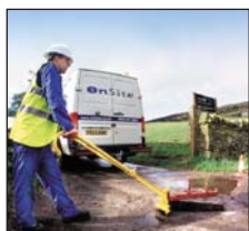
Gently push down on the handles to lift the cover
