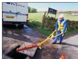
Slide the cover back on the Ezi-lift rollers
